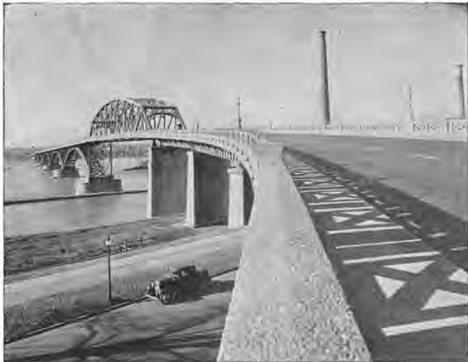
PEACE BRIDGE...WHICH LINKS THE U. S. AND CANADA
